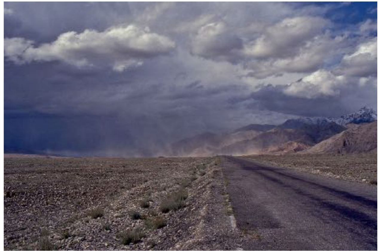
Karakoram Highway, near Kashi, far western China
