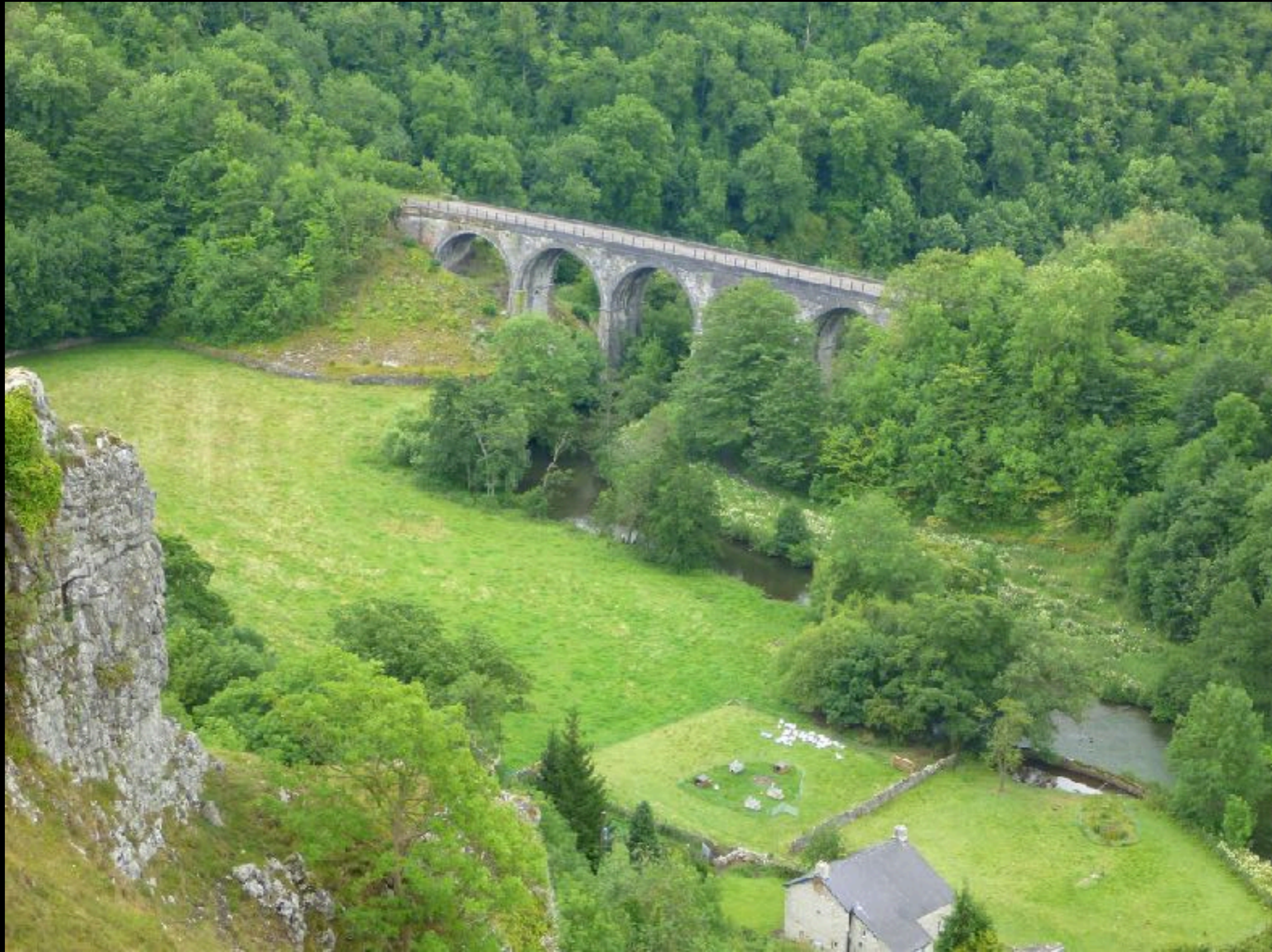
Headstone viaduct, Derbyshire 2011
